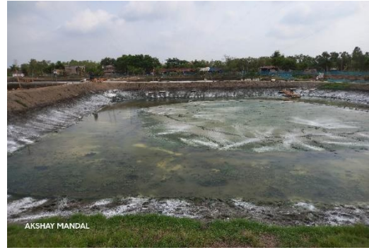
Fig-2: Application of lime on the pond bottom
